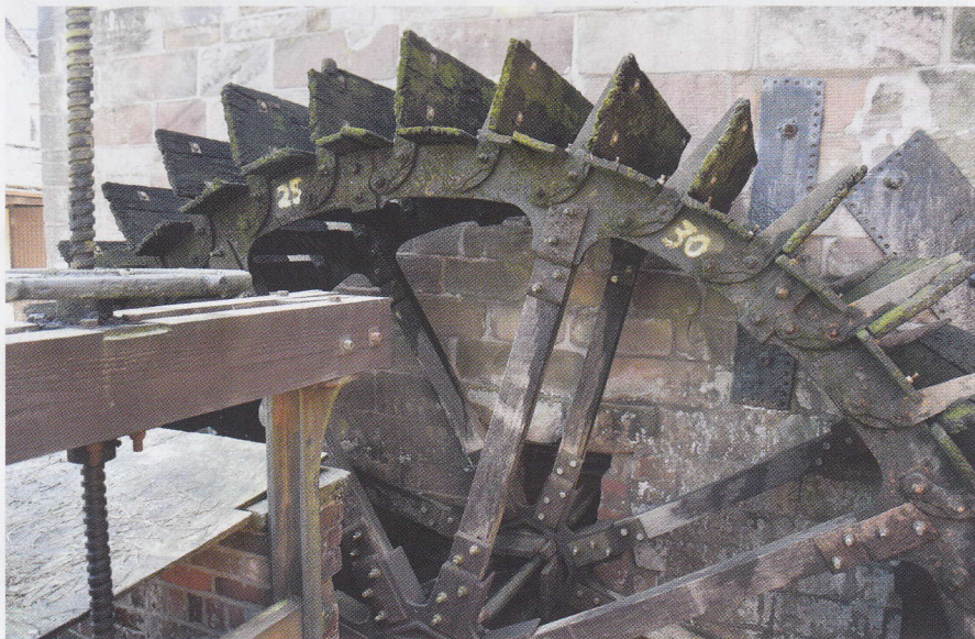
The all-important waterwheel. When in gear and with a normal head of water, it turns at around five revolutions per minute.
